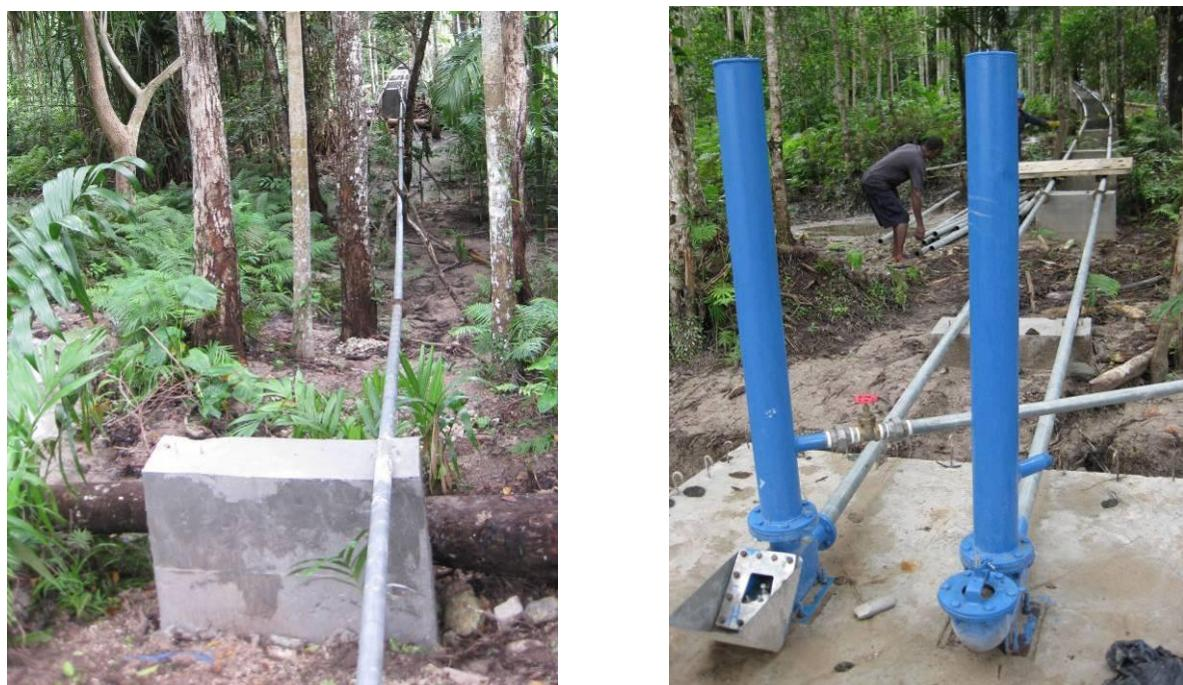
Figure 23: Drive pipes and supports
