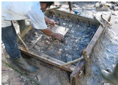
Figure 7: Construction of pump basement, NTT
