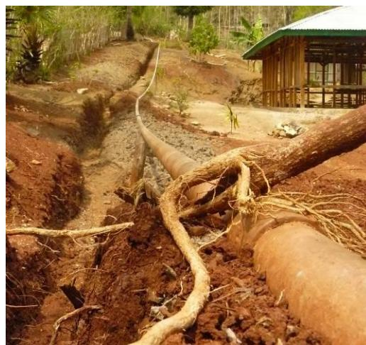
Figure 21: Burring delivery pipe
