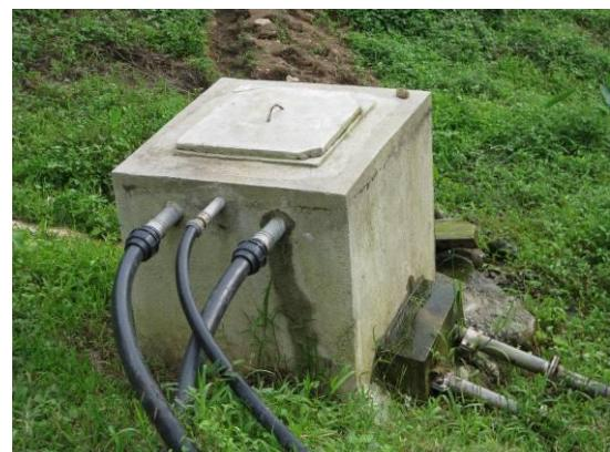
Figure 5.a: Header tank for 6 pumps from AID Foundation
