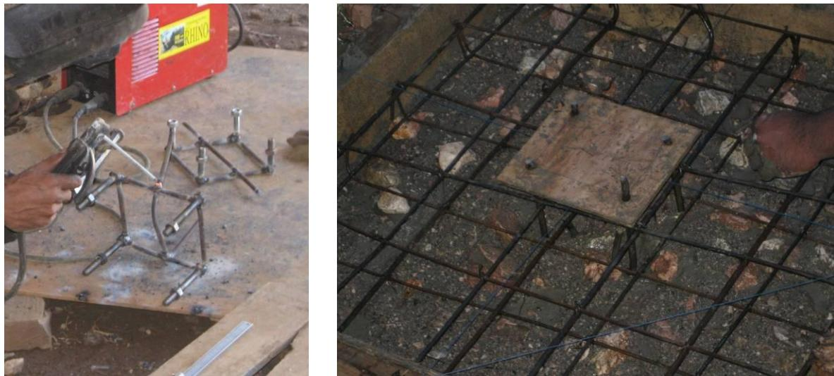
Figure 22: Construction of the pump basement
