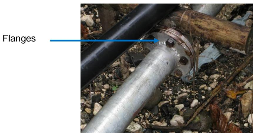
Figure 6: Drive pipe and flanges
