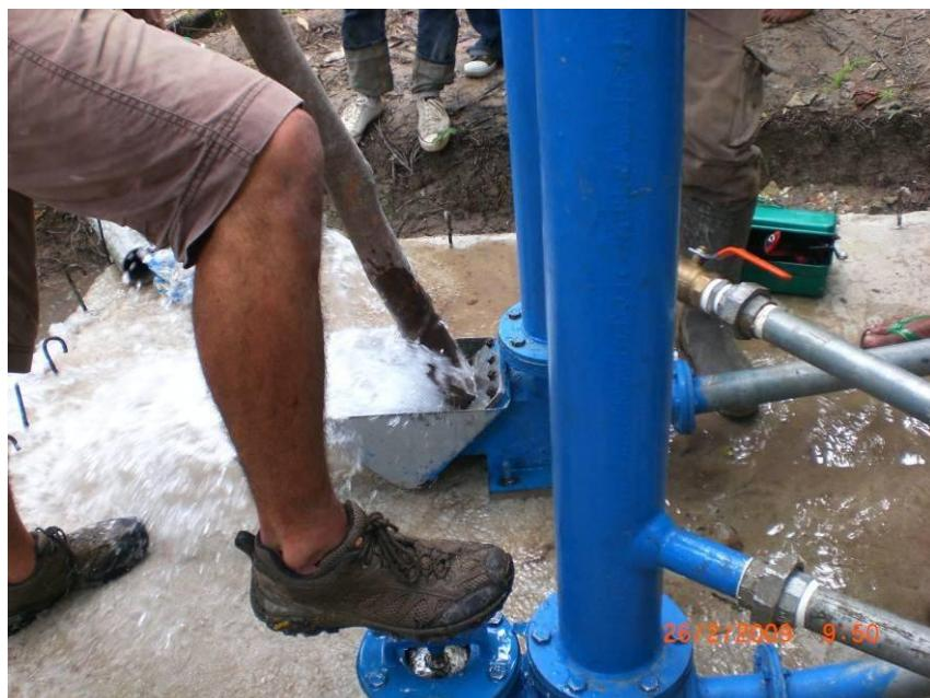
Figure 26: Priming the Hydraulic Ram Pump
